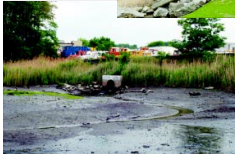
The contaminants that are generated on land find their way to bays, beaches and harbors through storm water outfall pipes like this one, pictured upper right. Outfalls tend to be hidden but the contaminants they discharge result in serious impacts to our special places along the coast. Photos courtesy of Eileen Keenan
